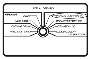
To return to auto mode, bring **parameter knob** to the MANUAL OVERRIDE position. The value of the desired position will flash, then press the **push button** to switch back to auto mode.
