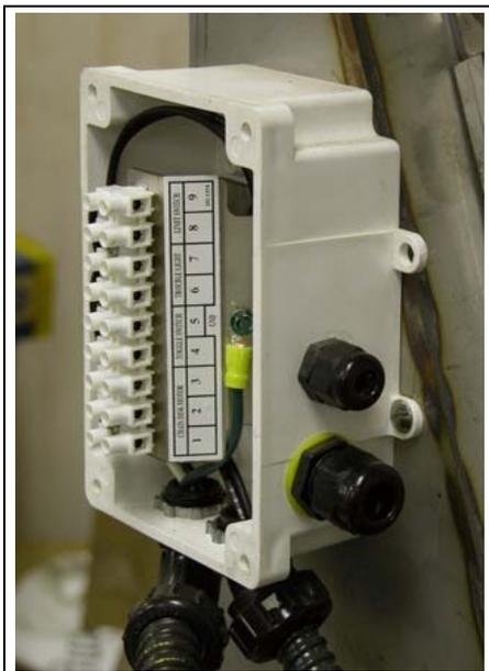
Fig. 10-A Chain Disk Junction Box
