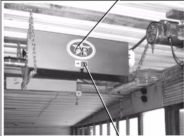
DC-996 is located on the front cover of the drive unit.
