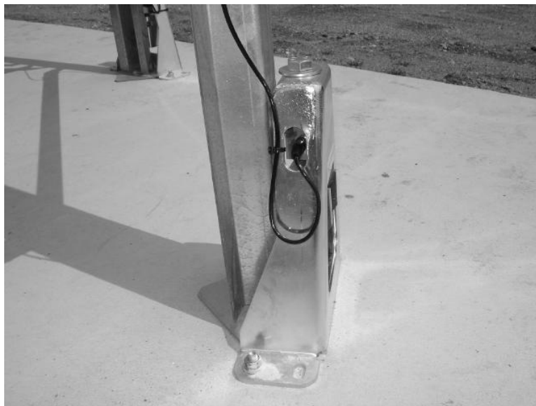
FIGURE 1: A FINISHED 'A' FRAME INSTALLATION
