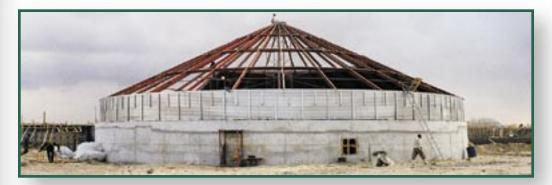
high ribs. They are reinforced with structured steel roof trusses on all 40-foot diameter bins and larger. VAL-CO's structural roof system is rated for 12,000 pounds of peak load. Top side wall sheets bolt directly to roof trusses for a more secure roof/wall joint.
