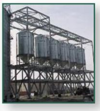
At the base of every hopper tank you will find a structural system of steel wide flange support columns designed to provide maximum strength. The support base is bolted into concrete while the top of the beam is double bolted to the tank compression ring. Designing the right slope is critical to your operational success. We offer 45° and 60° hoppers to accommodate your applications.
