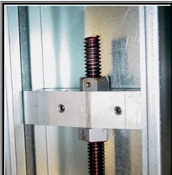
Figure 8 – Install New Load Block
