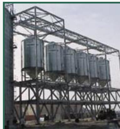
At the base of every hopper tank you will find a structural system of steel wide flange support columns designed to provide maximum strength. The support base is bolted into concrete while the top of the beam is double bolted to the tank compression ring. Designing the right slope is critical to your operational success. We offer 45° and 60° hoppers to accommodate your applications.
