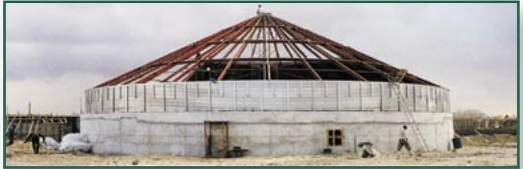
high ribs. They are reinforced with structured steel roof trusses on all 40-foot diameter bins and larger. VAL-CO's structural roof system is rated for 12,000 pounds of peak load. Top side wall sheets bolt directly to roof trusses for a more secure roof/wall joint.
